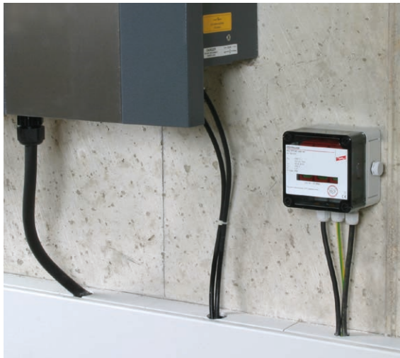
Figure 16 DEHNcube YPV SCI 1000 1M type 2 arrester for protecting inverters (1 MPPT)
