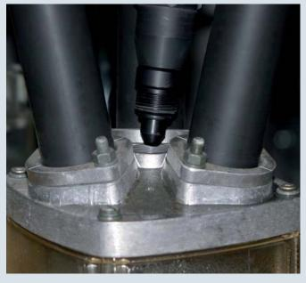
Screwing a special screw plug into a cable sealing end using an angled operating head
