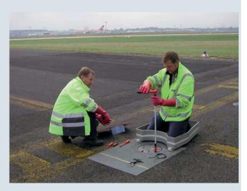
The insulating extension is used as insulating intermediate section when attaching the illuminant.
