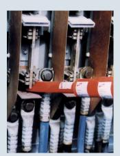
Chamfered flat cleaning head in use
