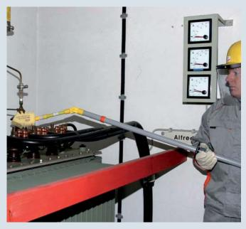
Damp cleaning of a transformer using the FRS ZK MS damp cleaning kit
