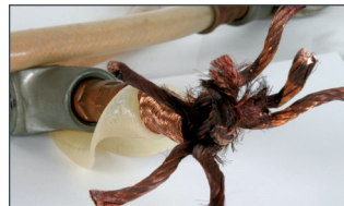
Approx. 30 year old device with a reduced cable cross-section as a result of copper corrosion.
