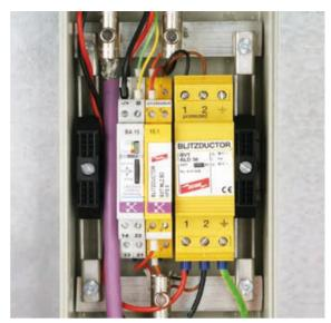
Figure 9.16.10 Protection of wind measurement equipment (anemometer)
