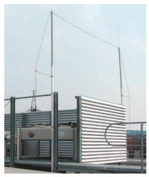
Figure 5.1.8.13 Isolated air-termination system with DEHNiso Combi
