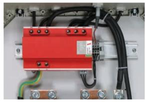
Figure 9.18.8 DEHNlimit PV 1000 V2 spark-gap-based type 1 combined arrester
