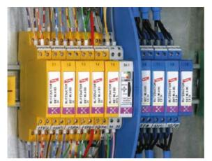
Figure 8.2.6.3 Monitoring of surge protective devices by means of the DRC MCM XT condition monitoring unit
