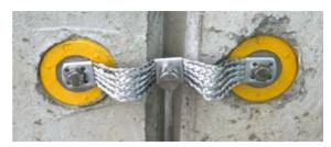
Figure 5.5.2.8 Bridging braid with fixed earthing terminals
