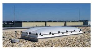
Figure 5.1.1.17 Protection of small-sized roof-mounted structures against direct lightning strikes by means of airtermination rods
