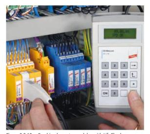
Figure 9.3.12 Combined arrester modules with LifeCheck
