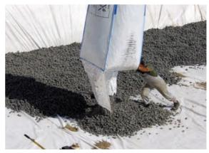
Figure 5.5.2.23 Perimeter insulation: Foam glass granulate is filled in; source: TECHNOpor Handels GmbH
