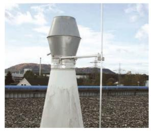
Figure 5.1.8.3 Air-termination rod with spacer
