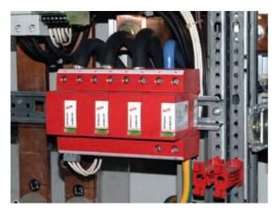
Figure 9.22.2 Lightning equipotential bonding by means of DEHNventil M
