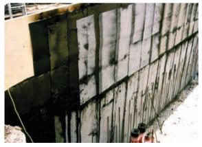
Figure 5.5.2.18 Bituminous sheetings used as sealing material
