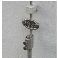
Figure 5.2.2.3.1 Test joint with number plate
