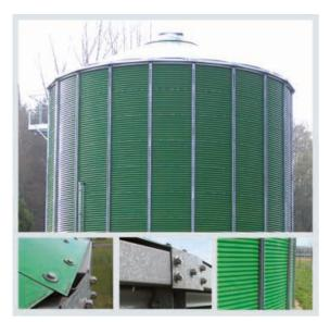
Figure 9.3.6 Fermenter made of bolted metal sheets
