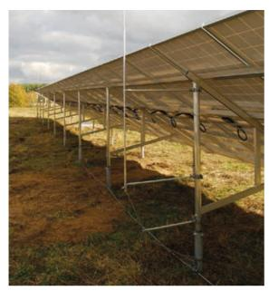
Figure 9.19.2 Lightning protection by means of DEHNiso spacers
