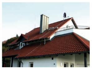
Figure 5.2.4.7 Protection of a residential building by means of DEHNcon-H (HVI light Conductor III)
