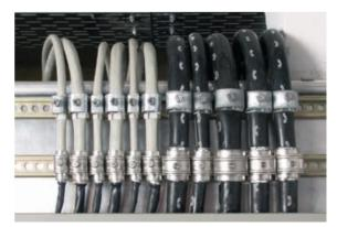
Figure 6.3.4 Lightning current carrying shield connection system (SAK)
