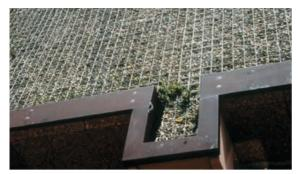
Figure 7.3.7a Galvanised reinforcement mats for shielding the building
