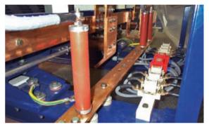
Figure 9.16.9 DEHNmid medium-voltage arresters installed in a transformer for wind turbines
