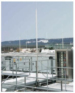
Figure 5.2.4.10 Installation of a HVI power Conductor
