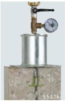
Figure 5.5.2.15 Wall bushing installed in the formwork
