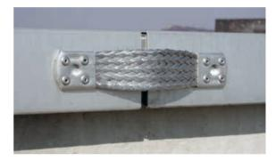
Figure 5.1.3.3 Bridging braid used for the roof parapet
