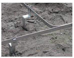
Figure 5.5.2.3 Foundation earth electrode
