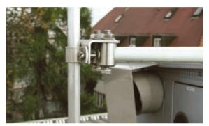
Figure 5.1.8.5 Supporting element for an air-termination rod
