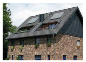
Figure 5.1.2.4 Building with photovoltaic system and sufficient separation distance; source: Blitzschutz Wettingfeld, Krefeld
