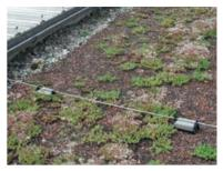
Figure 5.1.7.3 Conductor routing above the cover layer
