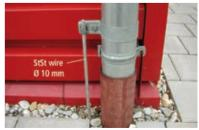
Figure 5.2.2.1.4 Earth connection of a downpipe
