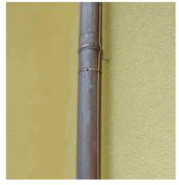
Figure 5.2.2.2.4 Down conductor installed along a downpipe
