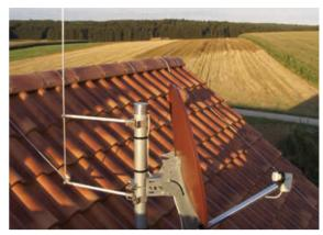
Figure 5.1.2.5 Antenna with air-termination rod and spacer
