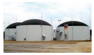
Figure 5.2.4.18 Protection of a biogas fermenter by means of a HVI Conductor
