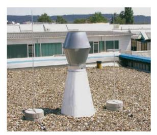
Figure 5.1.8.2 Isolated air-termination system – Protection by an air-termination rod
