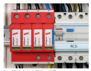
Figure 7.8.1.2 Multipole DEHNguard M TT surge arrester
