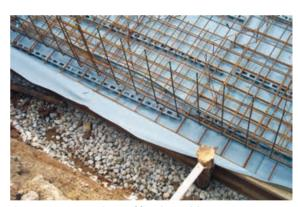
Figure 5.5.2.10 Membrane of foundation slabs
