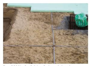
Figure 5.5.2.21 Detailed view of a ring earth electrode; source: Company Mauermann
