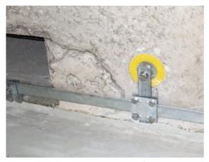
Figure 7.7.1.1 Ring equipotential bonding and fixed earthing terminal for the connection of metal installations
