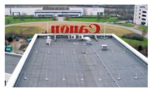
Figure 5.1.8.9 Elevated air-termination system; source: Blitzschutz Wettingfeld, Krefeld
