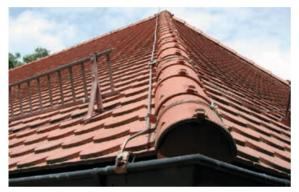
Figure 5.1.1.18 Gable roof with conductor holder
