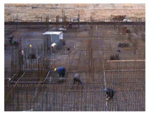
Figure 5.5.2.6 Meshed foundation earth electrode
