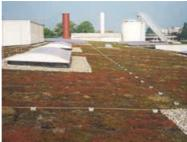
Figure 5.1.7.2 Air-termination system on a green roof
