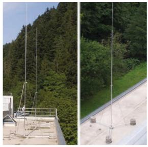
Figure 5.1.11.1 Protection against direct lightning strikes by means of self-supporting air-termination rods
