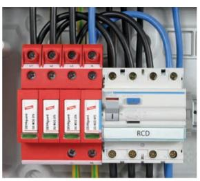
Figure 7.7.2.3 Multipole DEHNguard M TT surge arrester
