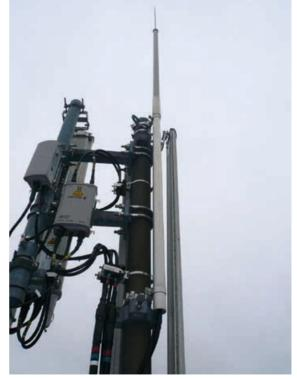
Figure 5.2.4.14 HVI Conductor installed on a radio tower
