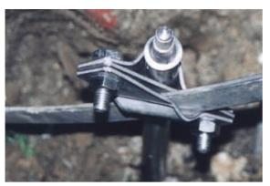
Figure 5.9.4 Connection of an earth rod to the ring earth electrode of the station
