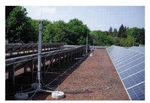
Figure 5.2.4.5 Protection of a PV system by means of a HVI light Conductor
