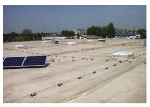
Figure 5.1.3.2 Practical use of air-termination rods
