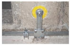
Figure 7.4.3 Connection of the ring equipotential bonding bar to the equipotential bonding network via a fixed earthing terminal
