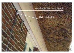
Figure 5.1.5.7 HVI Conductor led through the fascia board
