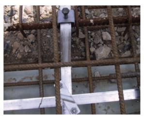
Figure 5.5.2.4 Foundation earth electrode in use
