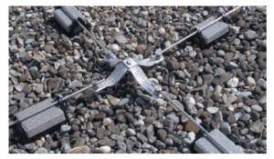
Figure 5.4.1.1 Air-termination system – Expansion compensation by means of a bridging braid
