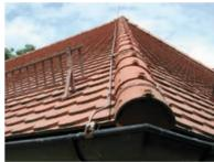
Figure 5.2.2.1.3 Air-termination system connected to the gutter
