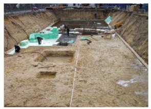
Figure 5.5.2.20 Ring earth electrode in case of perimeter insulation; source: Company Mauermann
