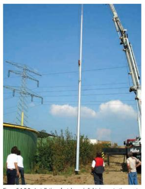
Figure 5.1.8.8 Installation of a telescopic lightning protection mast
