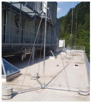
Figure 5.1.8.7 Isolated air-termination system for roof-mounted structures
