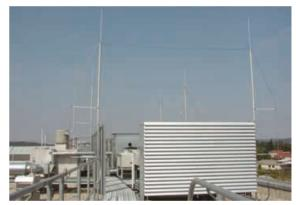
Figure 5.1.8.11 Isolated air-termination system with DEHNiso Combi
