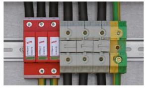
Figure 9.16.7 Protection of the stator side of the generator
