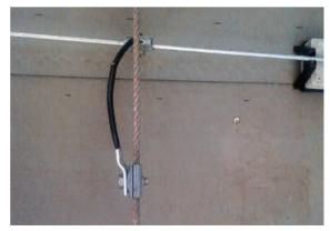
Figure 5.1.12.2 Incorrect installation: Safety rope system intersects the air-termination system
