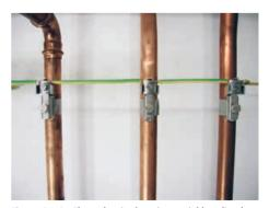
Figure 6.1.6 Through-wired equipotential bonding bar
