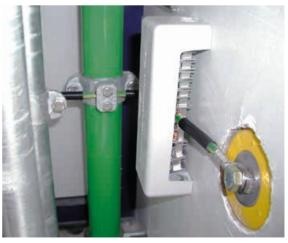
Figure 7.5.1.1 Connection of the EBB to the fixed earthing terminal
