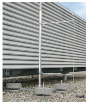
Figure 5.1.8.10 Tripod for isolated supporting tubes
