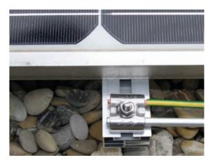
Figure 9.18.3 UNI earthing clamp: A stainless steel intermediate element prevents contact corrosion, thus establishing reliable long-term connections between different conductor materials
