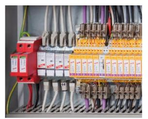
Figure 9.16.11 Example of surge protective devices in a pitch system
