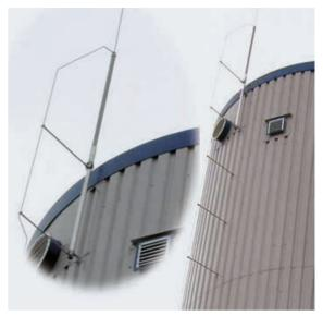
Figure 9.3.7 Protection of a fermenter made of metal sheets by means of an isolated air-termination system (source: Büro für Technik, Hösbach)
