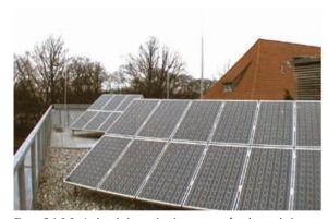
Figure 5.1.8.6 Isolated air-termination system of a photovoltaic system
