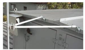
Figure 5.1.8.4 Angled support for an air-termination rod
