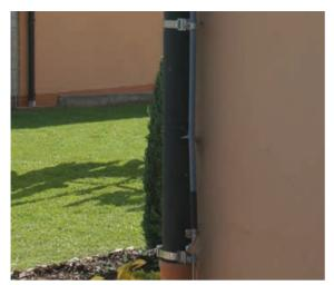
Figure 5.2.4.6 Connection of DEHNcon-H (HVI light Conductor I) to the earth-termination system
