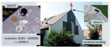
Figure 5.1.4.2 Example of damage: Sheet metal
