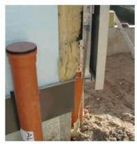
Figure 5.2.2.3. Earth connection of a metal façade
