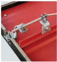
Figure 5.1.4.6 Sample construction on a standing seam roof
