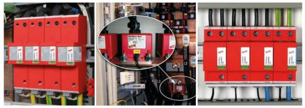
Figure 7.5.2.9 Lightning current arrester at the transition from LPZ 0<sub>A</sub> to LPZ 1
