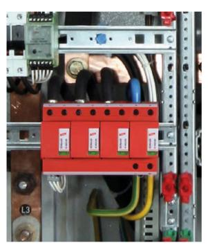
Figure 6.2.2 DEHNventil combined arrester for installation in conformity with the lightning protection zone concept at the boundaries from  $0_A$ –2
