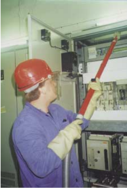
Figure 11: Cleaning of the frame of LV switchgear
