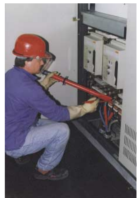
Figure 10: Cleaning of LV switchgear applying the methods (5.1 + 5.2)
