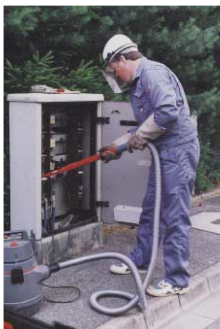
Figure 9: Cleaning of a low-voltage cable distribution board
