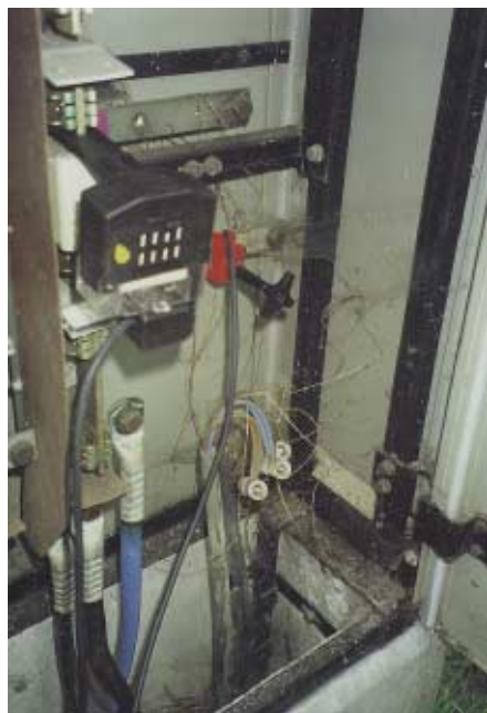
Figure 5: cable distribution before cleaning
