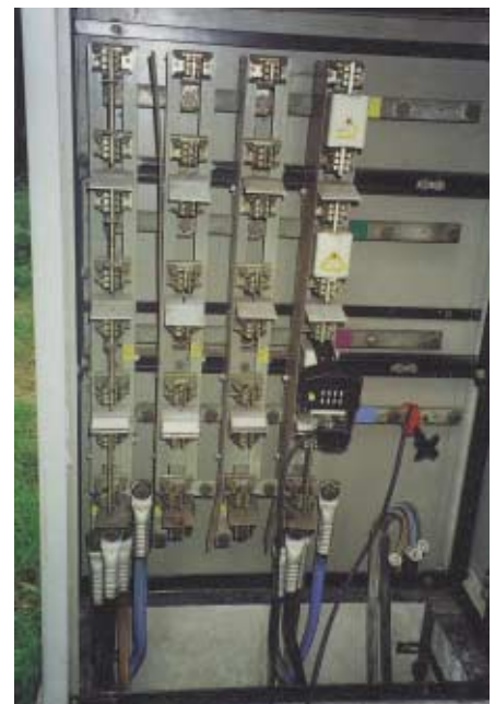
Figure 6: cable distribution after cleaning
