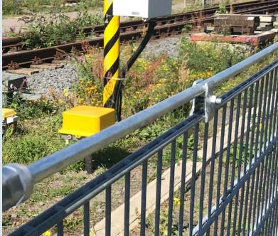
Short-circuit wire on a gabion or grating fence
