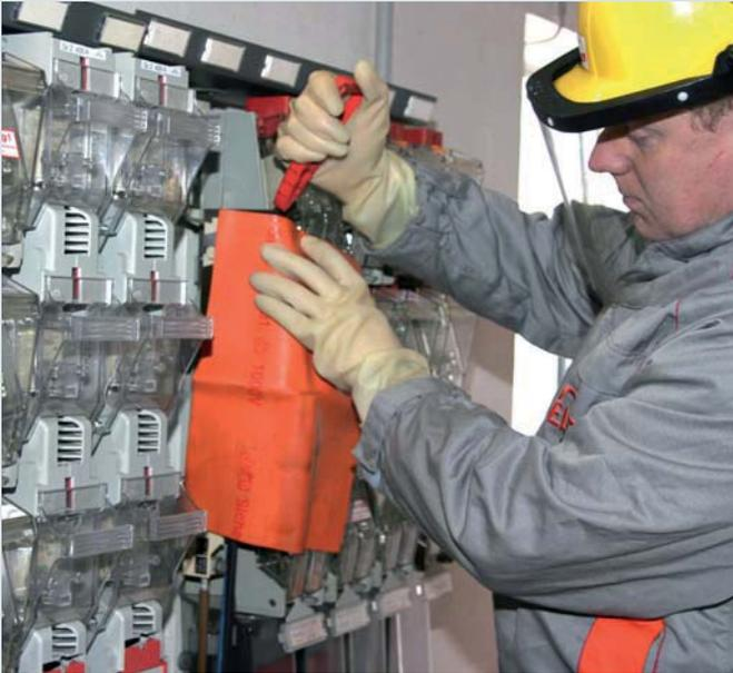
Live working with insulating gloves up to 1000 V
