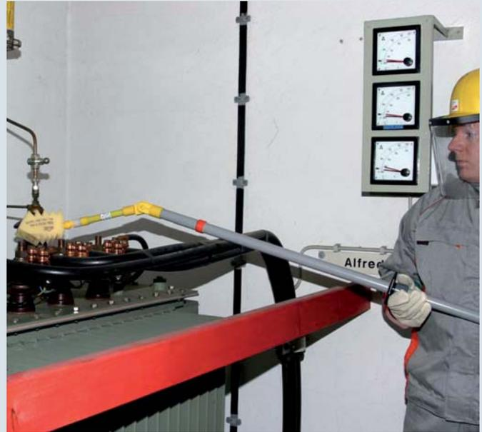
Damp cleaning of a transformer using the FRS ZK MS damp cleaning kit
