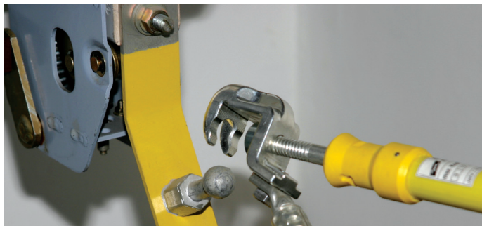
Installation of an earthing and short-circuiting device with universal clamp for fixed ball points (20 or 25 mm)
