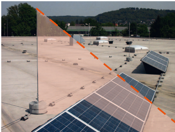
Figure 11 Determination of the protected zone using the protective angle method
