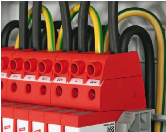
Figure 7 Simple series connection by means of a STAK 25 terminal
